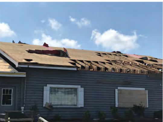
Figure 18: Commercial structure in Interior Panama City Sustaining severe wind damage.
