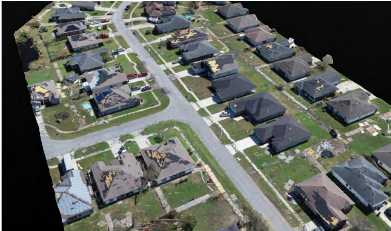
Figure 8: Preliminary 3D model of a portion of the Cedar Crossing subdivision, created using Structure from Motion photogrammetry.
