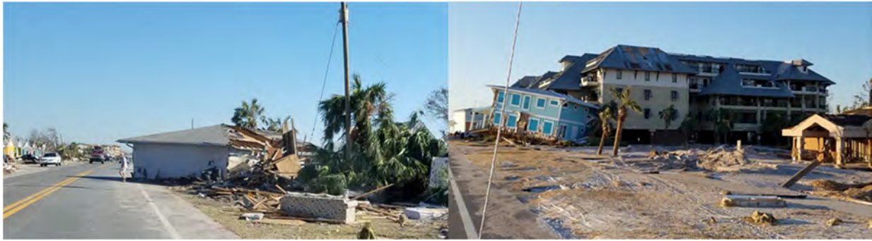
Figure 29: (left) Home pushed on to US-98 by storm surge; (right) Home pushed into multi-family residential complex by storm surge in Mexico Beach.
