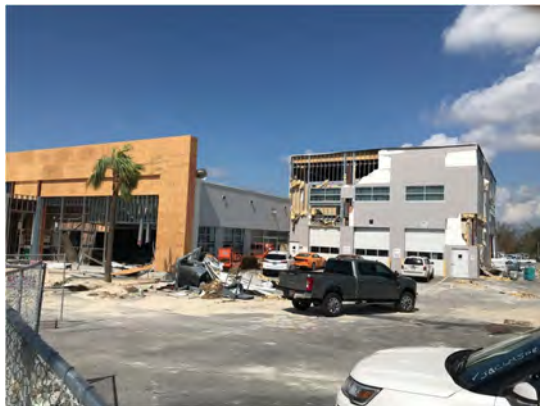
Figure 17: Commercial structure in Interior Panama City Sustaining moderate wind damage.
