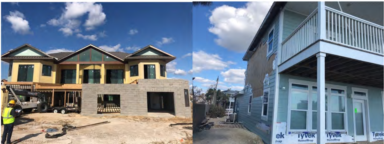
Figure 28: Newer buildings with minor damage in Mexico Beach.
