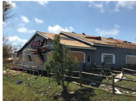
Figure 18: Commercial structure in Interior Panama City Sustaining severe wind damage.
