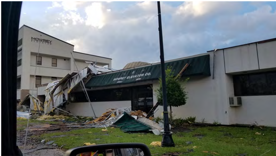
Figure 43. Commercial building (Mowrey Elevators) sustaining severe roof damage on Lafayette St. in Marianna.
