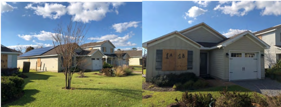
Figure 38: Residential structure in Port. St. Joe with solar panels intact (left) and minor vinyl soffit damage to front elevation (right), windows were covered with plywood.
